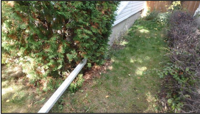
5. Improper slope or drainage
