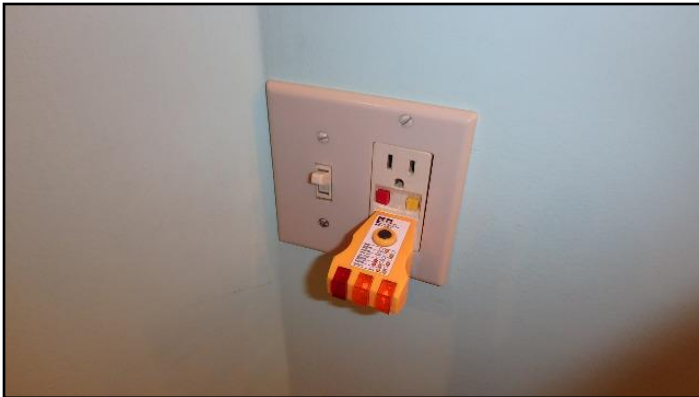
14. Test faulty on GFCI/GFI (Ground Fault..
