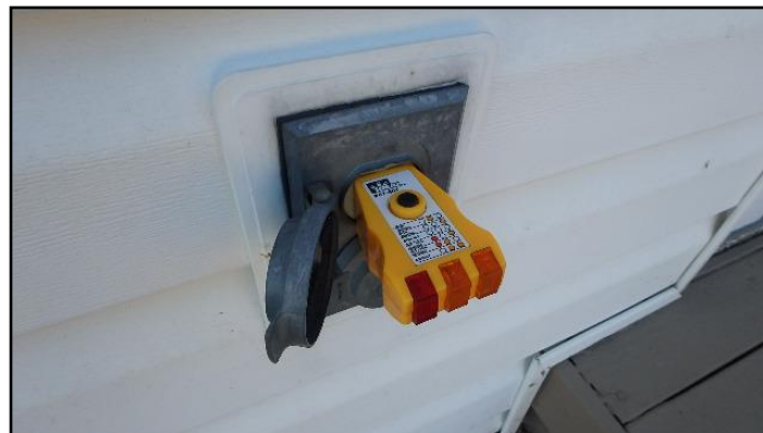
13. No Ground Fault Circuit (GFCI)
